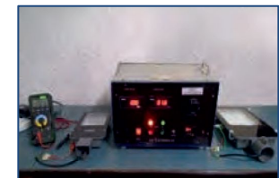
HV Test + Insulation
