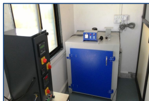
Temperature Controlled oven
